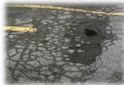
*Repairing cracks in pavement prevents pollutants from accumulating in lot.*
